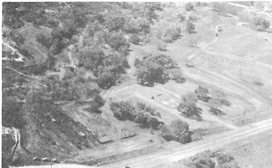
LOOKING DOWN ON THE SITE FOR THE BIG NEW $125,000 TRAILER PARK THAT JOHN M. JONES AND SON ARE RUSHING TO COMPLETION. PHOTO TAKEN BY CLARKE IRVINE.
